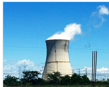
Davis–Besse Nuclear Power Station's cooling tower in July 2015
