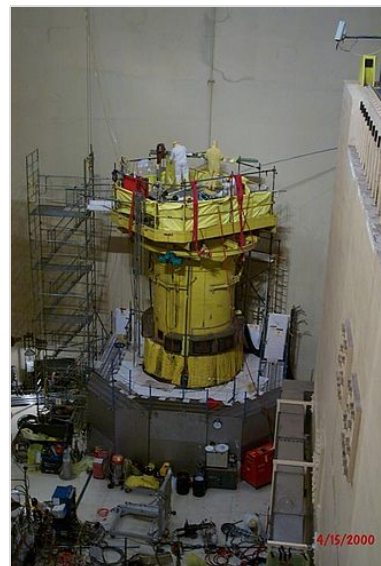
The reactor head under inspection
